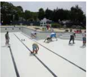
Pool Being Re-plastered
