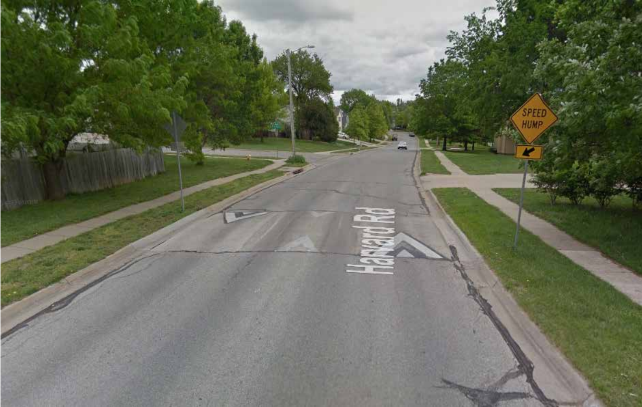
Speed cushion just west of the intersection of Harvard Rd and Eldridge St.
